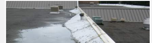
Roofs would be repaired or replaced
