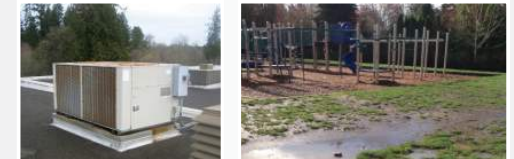
HVAC and drainage would be addressed
